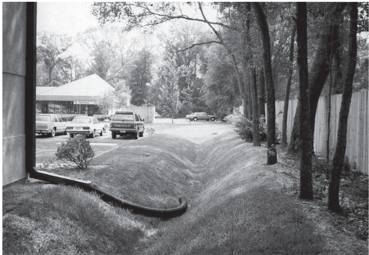
Infiltration Practice: Directing root to grassed areas.
